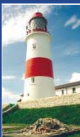
The photograph used on this issue's cover is of Souter Lighthouse, Sunderland
